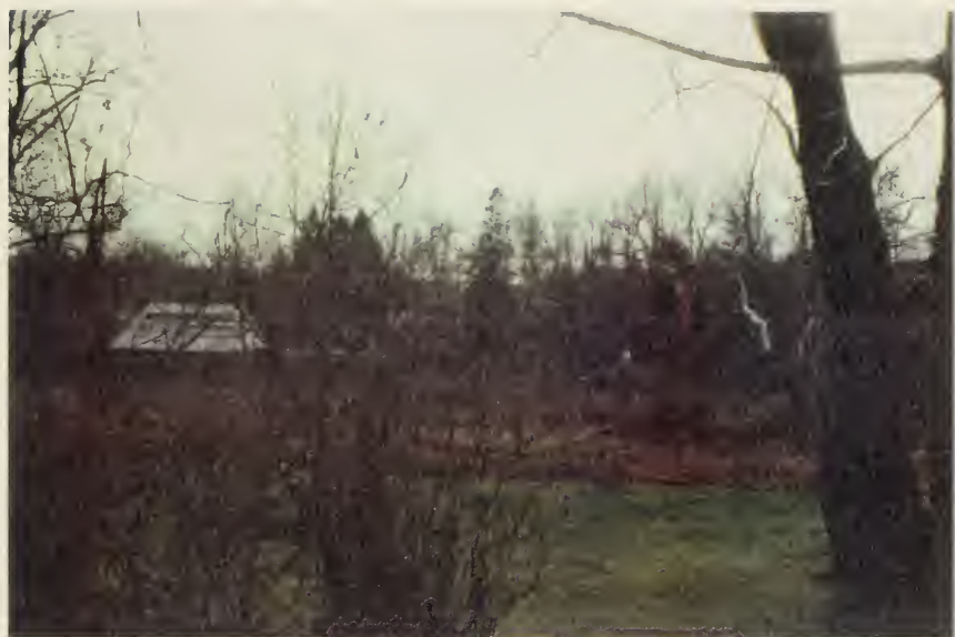
Fig. 119 The Yellow Springs pool house and gazebo with a view of the overgrown, surrounding vegetation. Photograph by the author, 1995.
